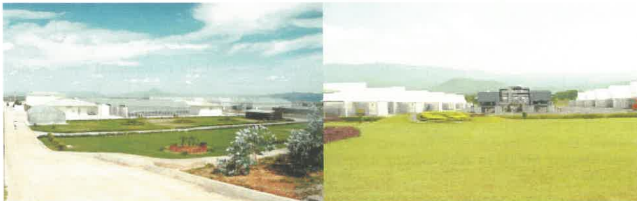
TECHNITUBER® Production Facility, Manpura, India
